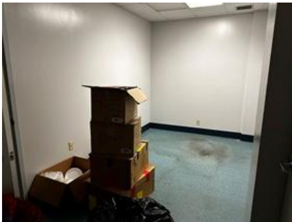
Interior View of Subject Property
