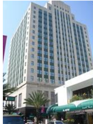
Lease 2 Alfred I. Dupont Building
